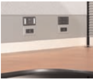
Quad power and data combination tile above worksurface height.
