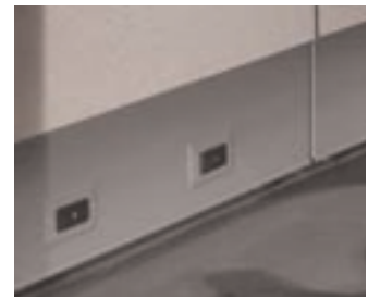
Dual power tile at raceway height
